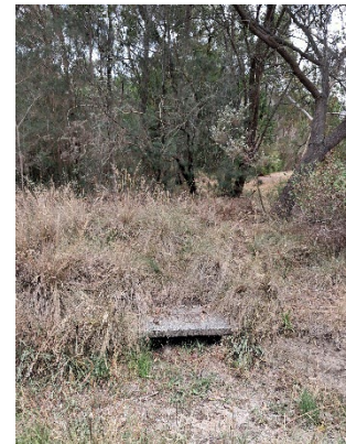
Side entry pit on Bayview Road
