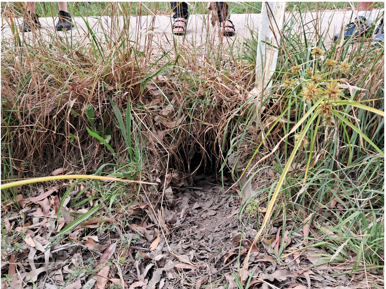
Figure 4. Outlet from Foam Street to the foreshore, which will need upgrading to cope with climate change.
