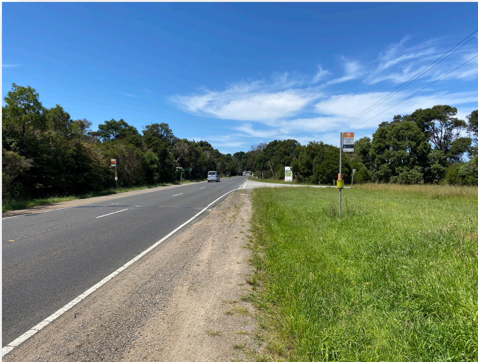
Figure 4: Frankston-Flinders Rd at Merricks Beach Rd: Typical View
