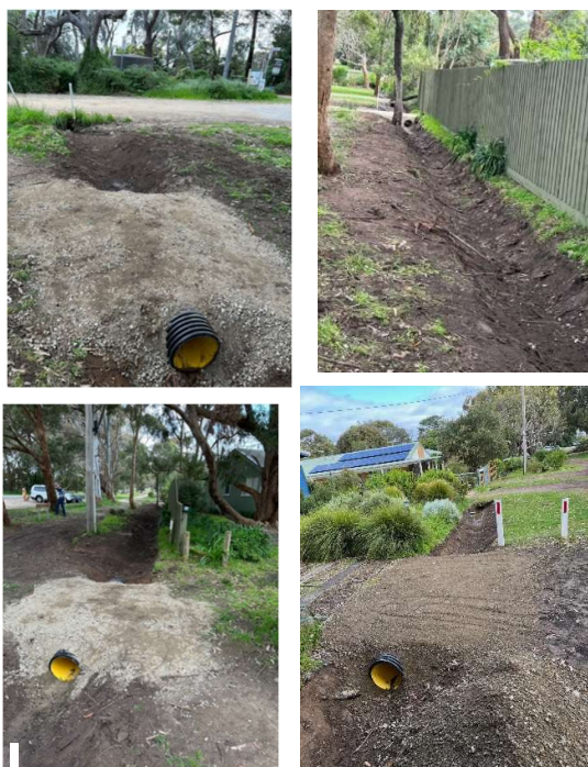
MB Rd Works in progress
